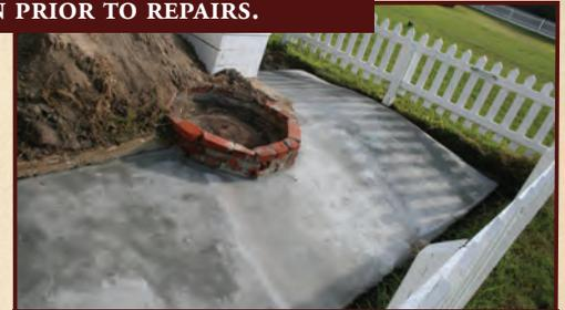
**THE COMPLETED CISTERN TOP IS "CURED" BEFORE IT IS COVERED WITH NEW SOD FOR PROTECTION FROM THE ELEMENTS.**
